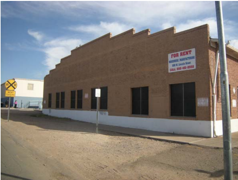
Photo 1. View of original 1927 building from intersection of 9 th Avenue and Lincoln Street, looking northeast.
