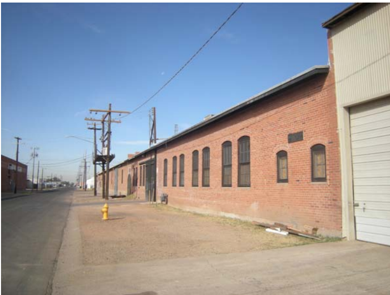
Photo 3. View of 1943 addition from Lincoln Street, near 7 th Avenue, looking west. Original 1927 building is in background.
