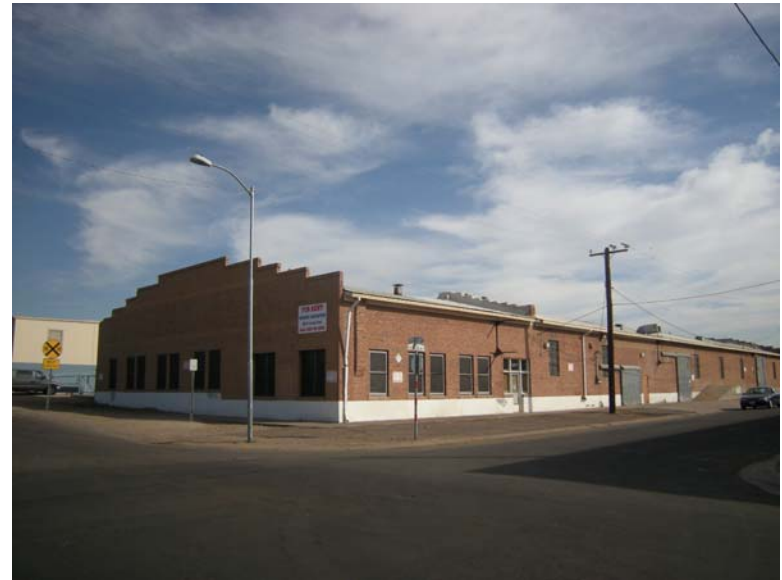
Photo 2. View of original 1927 building from opposite corner of 9 th Avenue and Lincoln Street, looking northeast.
